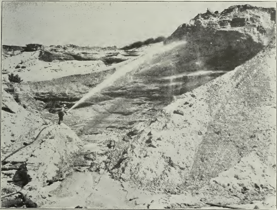
Fig. 21. Hydraulic quarrying of the St. Peter sand. The sump and pump are just beyond the left foreground of the picture. (Photograph by courtesy of Ottawa Silica Company.)
